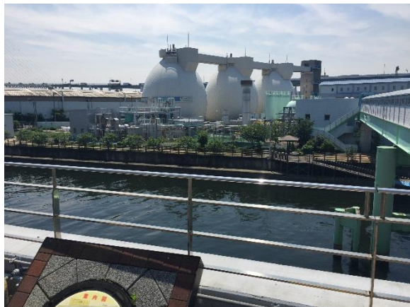
On the left are three anaerobic egg shape diagesters used to generate mentha. On the right, Mahound Al-Moaikel in the control room
