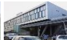
Doosan Power System India
