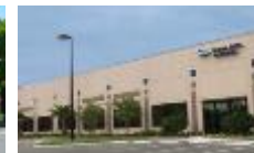
Doosan Hydro Technology
