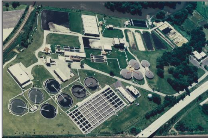
Fox Metro Water Reclamation Facility
