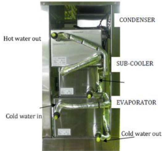
FIG 4 End view of unit showing water connections
