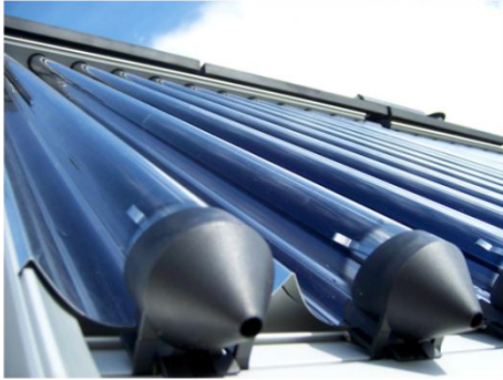
Close up of CPC (Compound Parabolic Concentrator) reflector
