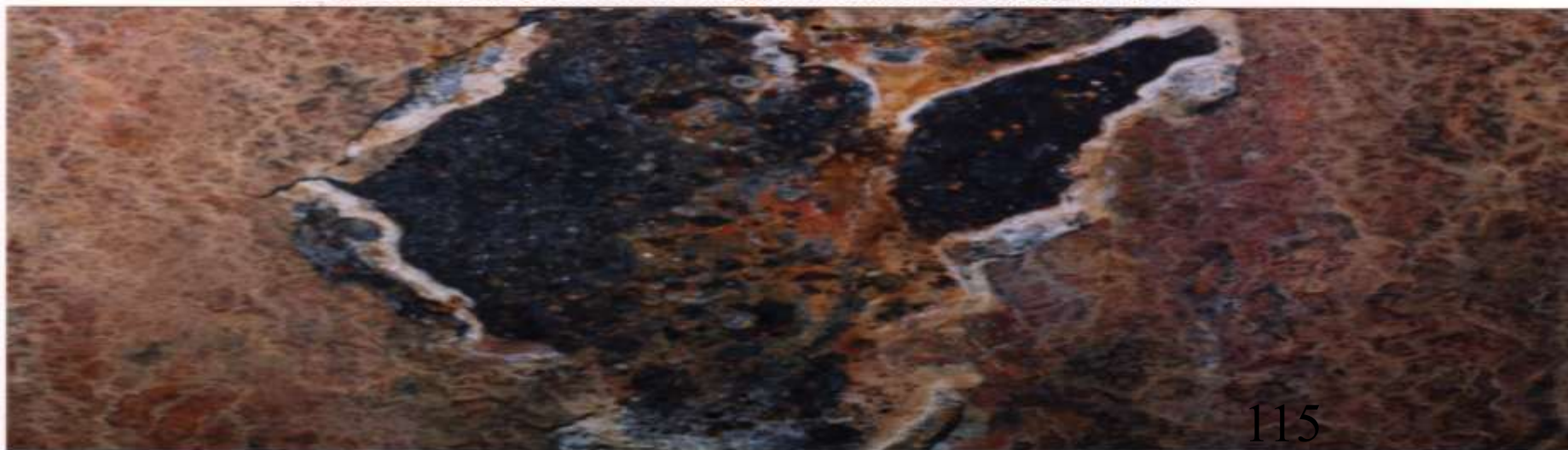
corrosion in the distillate tray
