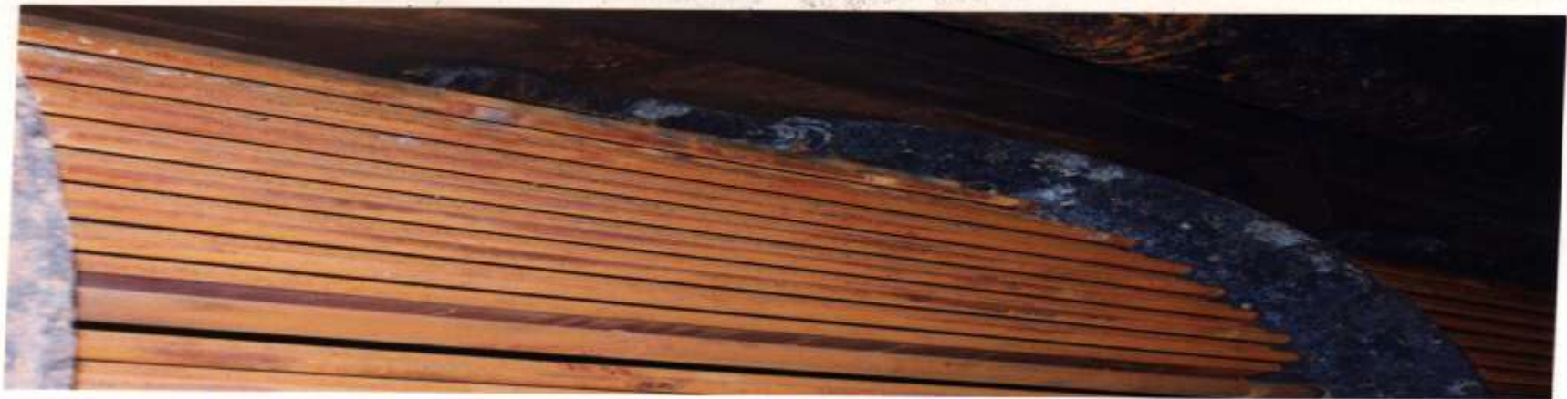
tube bundle tube supports roof plates and uncondensable extraction pipes
