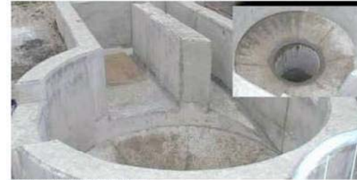
Civil construction and installation.
