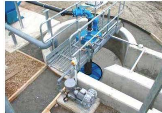
The completed Jetair installation.
