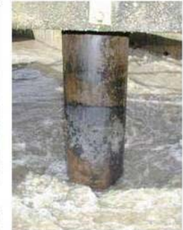
The effects of the continuous aeration can be clearly seen on the tank surface.
