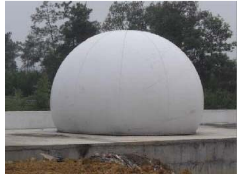
Biogas Storage Dome
